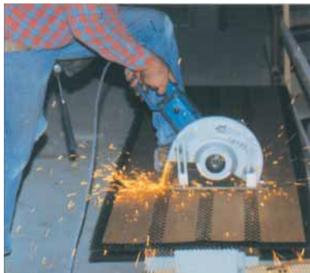
Cutting Secura Lath Sheets
