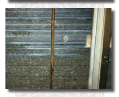
When a contractor has to form a concrete wall within a few inches of an existing structure, Stay-Form is an excellent product. By utilizing Stay-Form with rebar studs, hook ties, and a modular form system, a one-sided form or blindside wall can be constructed. If you do not have the luxury or room to strip formwork, Stay-Form is the right product for the job.
