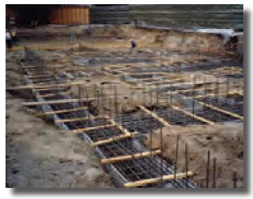
Grade beams are easily formed using Stay-Form and rebar or lumber as bracing. Some contractors prefer to backfill 75 to 90 percent up the grade beam prior to the concrete pour in order to minimize the required bracing. Backfilling acts as the bracing which will stop the formwork from spreading during the pour.
