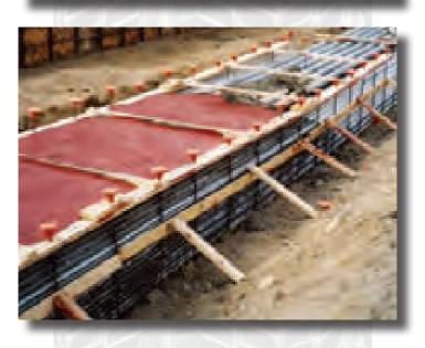
Electrical contractors find it easier to form ductbanks with Stay-Form than with plywood or conventional forming systems. The learning curve to train personnel how to install Stay-Form is quick, and the labor savings are significant due to the fact that form stripping is not necessary.
