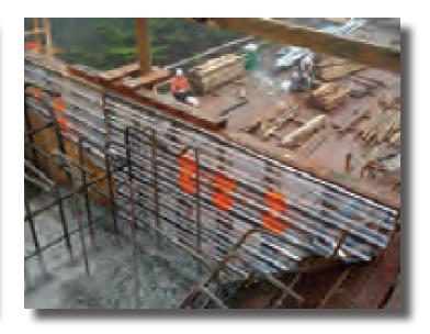
Contractors frequently use Stay-Form on bridge projects to form footings, edge forms and bulkheads. When building a cast-in-place segmental box girder bridge, forming the bulkheads has significant labor savings because the bulkhead does not have to be stripped.
