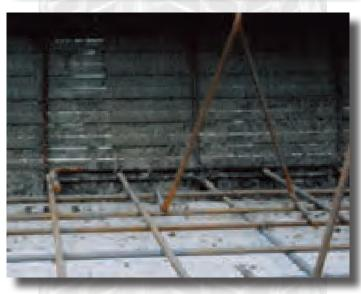
Stay-Form is an excellent product for forming bulkheads because it does not have to be stripped out after the concrete pour. (Plywood and modular forms have to be stripped.) There is also no scrabbling required in order to prepare the surface for the next pour.
