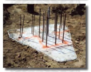
When forming below grade structures like a pile cap, Stay-Form can save a considerable amount of time and labor. You have no labor for stripping forms. If rebar or metal is used for bracing, it stays in place. (Wood bracing has to be removed.) Some contractors backfill around the Stay-Form prior to the pour therefore they minimize bracing and prevent a blowout of the form.
