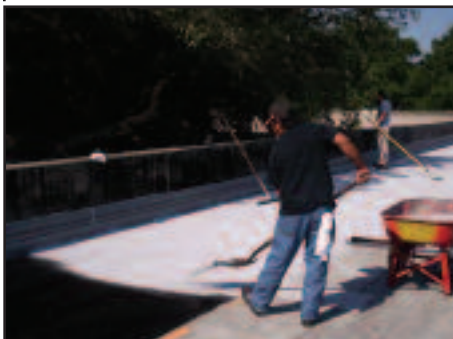
STEP 26: TOP SURFACE ARMORFLEX™ WITH EITHER: GRANULAR SURFACING
