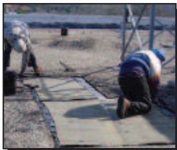
As a maintenance mastic
