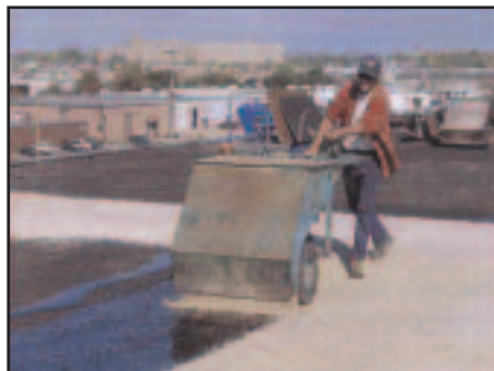
STEP 26: TOP SURFACE ARMORFLEX™ WITH EITHER: GRANULAR SURFACING
