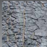
Alligatoring & Cracking
