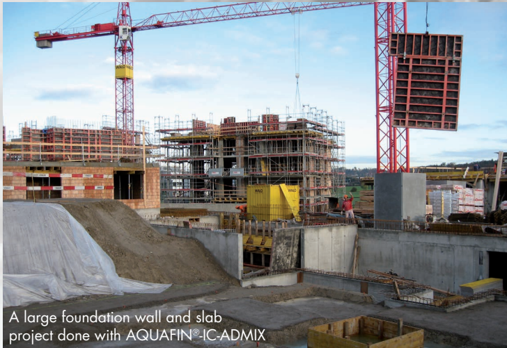
AQUAFIN®-IC-ADMIX added onsite and poured in Havre de Grace, MD
