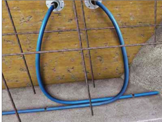
InjectPro-Hose installed using Nail Packers
