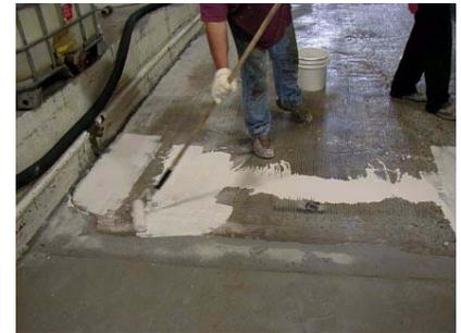
7. Pour appropriate amount of material onto slab and spread evenly with a roller or squeegee.
