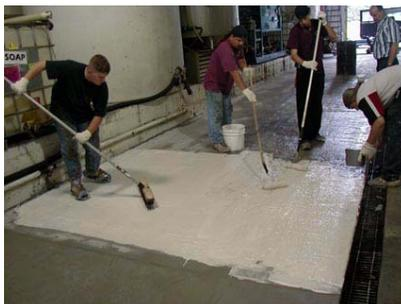
8. Carefully scrub SG2 into the pores with a long handled broom or scrub brush.
