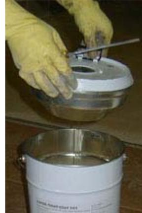
3. Completely drain Part B (hardener) into Part A (resin).
