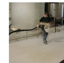
SG2 only: Application step 3: Broadcast #20 mesh (0.5 – 1.0 mm) sand to full rejection into fresh material.
