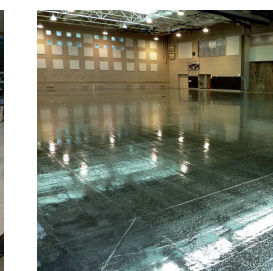
SG3: Finished installation ready to receive flooring and/or cementitious underlayment.
