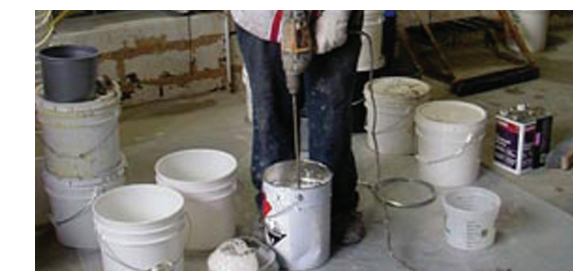
Mixing VAPORTIGHT COAT®-SG2 or -SG3 in supplied container.
