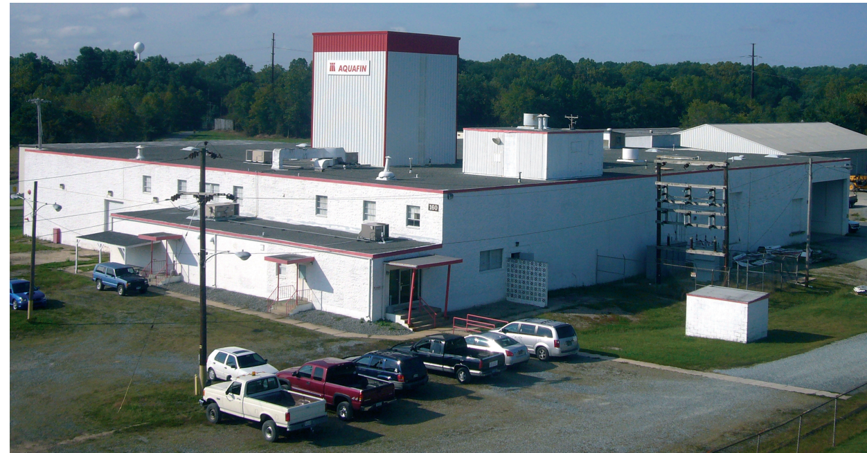
AQUAFIN Inc. plant in Elkton, MD, USA
