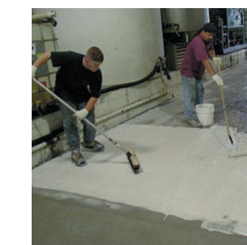
SG2: Application step 1: Scrub material into the substrate with a brush.
