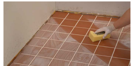
Use the ARDEX Sponge to cut through slurry
