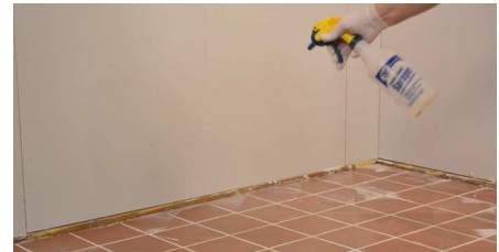
Spraying water on ARDEX WA
