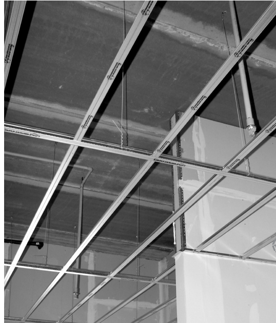
FrameAll Grid suspension system
