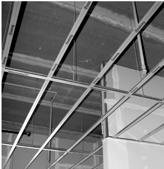
▲ Drywall Grid suspension system
