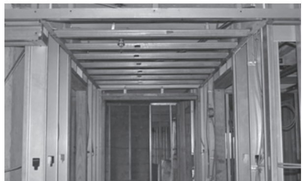
Corridor framing using traditional steel studs
