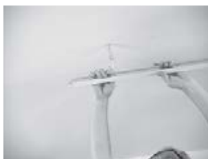
Install first main beam
