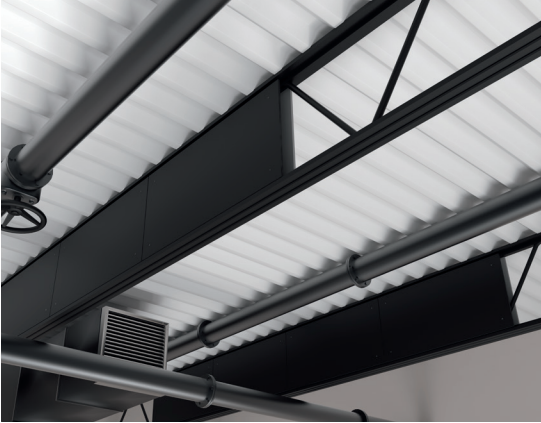
InvisAcoustics™ Panels in Black Truss Installation
