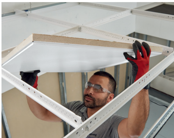
MetalWorks™ Tegular ceiling panel with Calla® 2820 acoustic infill panel – Total Acoustics™ ceiling system
