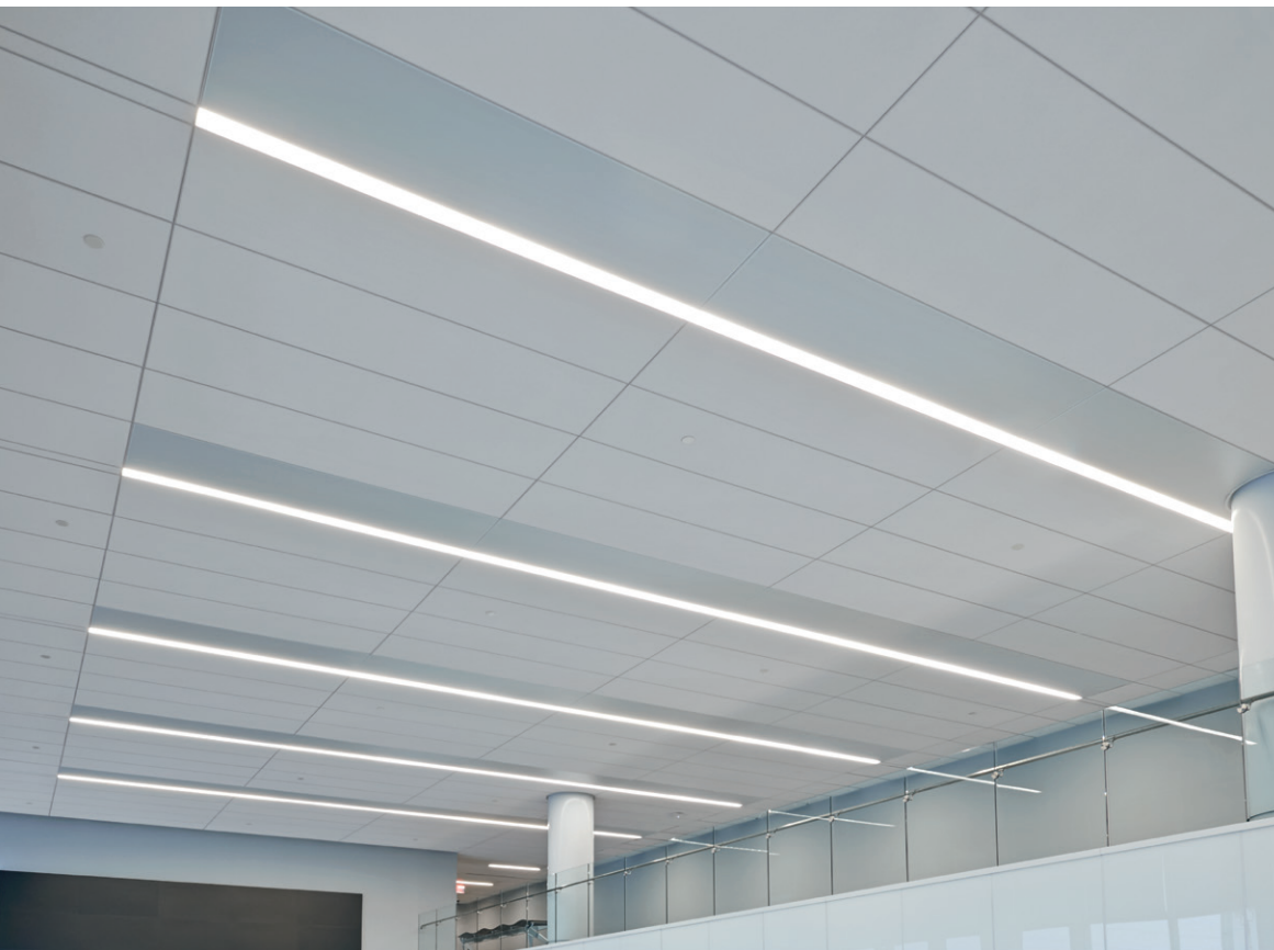
MetalWorks™ Tegular unperforated panels in White with Prelude® XL® 15/16® suspension system
