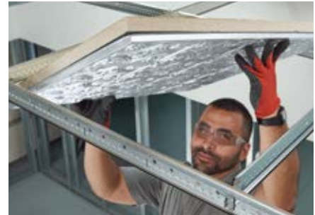
MetalWorks™ 3D Tin ceiling panel with Calla® 2820 acoustical infill panel – Total Acoustics™ ceiling system
