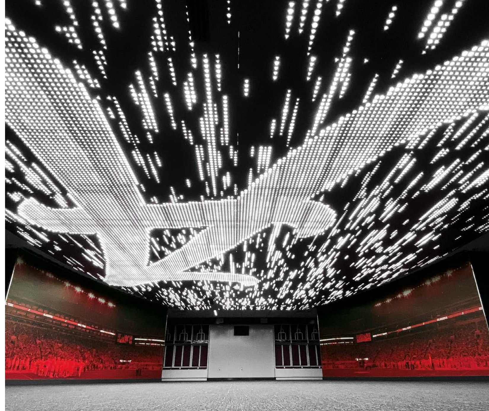
Custom MetalWorks Torsion Spring ceiling panels, University of Alabama Football Locker Room, Tuscaloosa, AL
