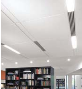
TechZone with Optima 48" x 48" panels on Interlude® XL 9/16" suspension system. CitiPlan, Chicago, IL
