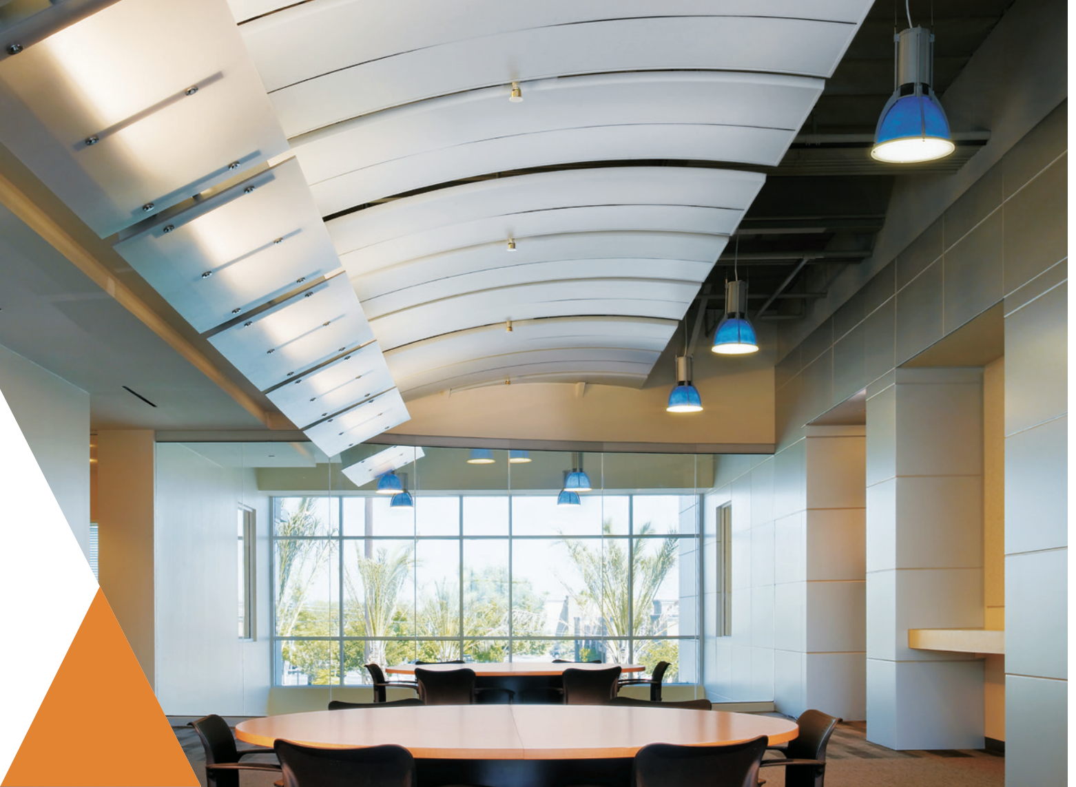
▲ Serpentina® Waves™ with R062 perforation in White; WLC Architects, Inc., Rancho Cucamonga, CA
