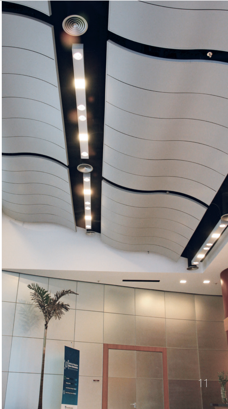
▼ Serpentina® Waves™ 8' x 12' unperforated Hill/Valley 45° arc in Silver Grey; Votorantim Bank, São Paulo, Brazil
