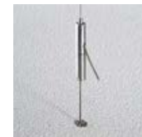
Embedded hardware in back of panel
