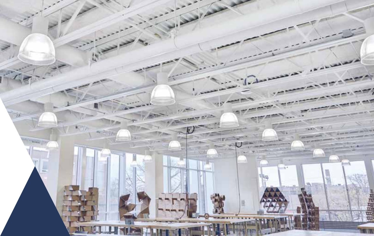
▲ Tectum Direct-Attach Ceiling Panels; Temple School of Architecture, Philadelphia, PA; NELSON, Philadelphia, PA
