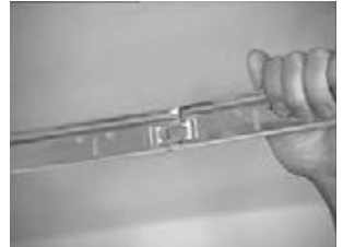
Join sections of main beam
