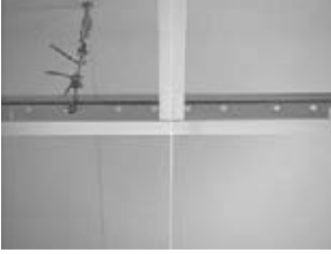
Align second guide string with first four-foot cross tee
