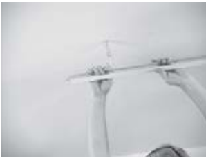
Install first main beam
