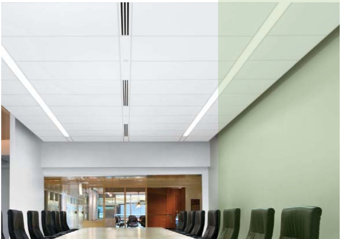
TechZone with Optima 48" x 48" panels and MetalWorks 6" x 48" technical panels on Suprafine XL 9/16" suspension system. American Society of Clinical Oncology, Alexandria, VA
