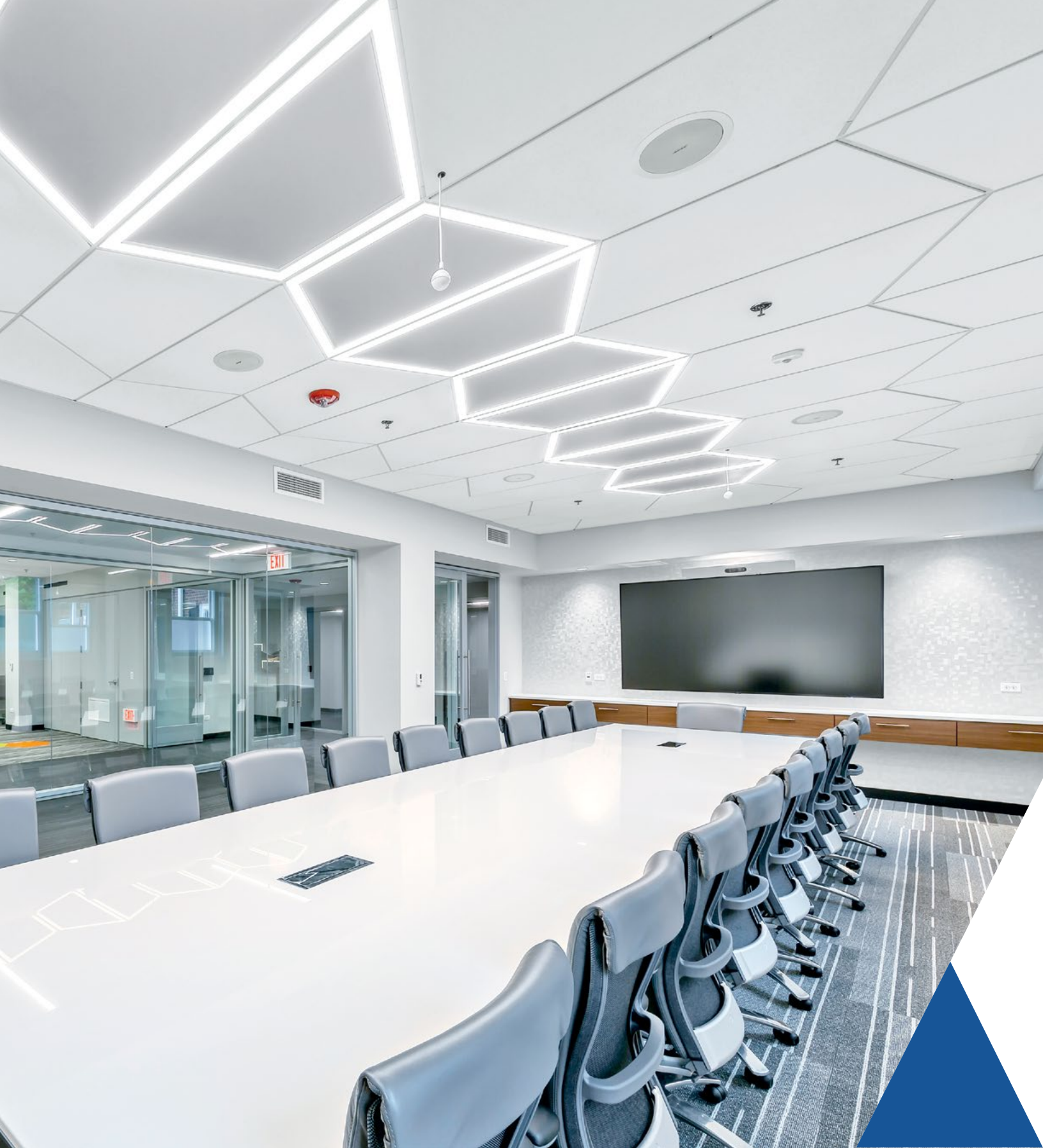
▲ ULTIMA® Shapes for DesignFlex® / MetalWorks™ Shapes for DesignFlex / SUPRAFINE® XM Suspension System, with Axis Sculpt Geometric Light Fixtures; Insurance Company Training Facility, Chicago, IL, The Interior Design Group, LTD
