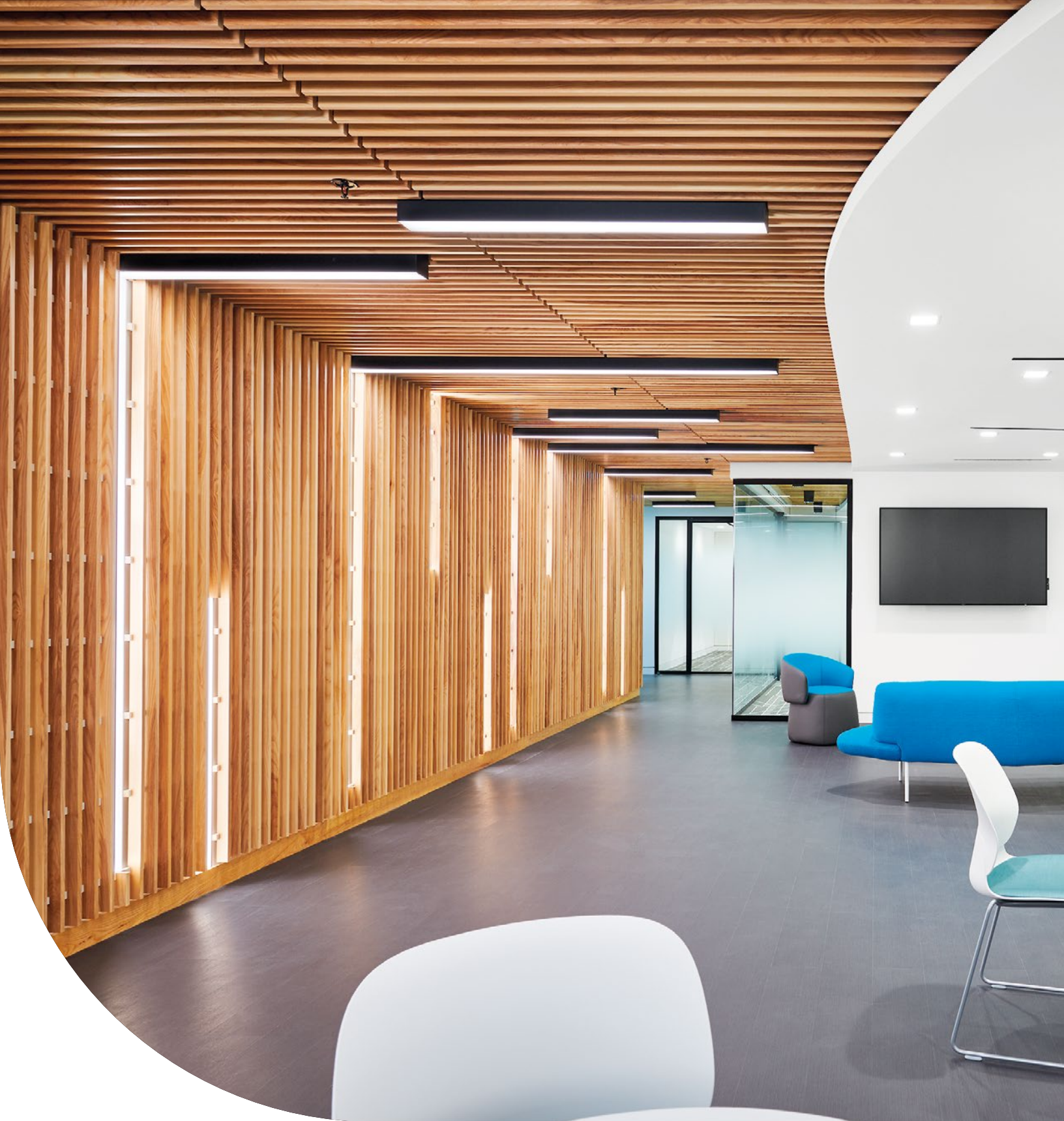
WoodWorks® ACGI Custom Grille, Federal Communications Commission Headquarters, Washington, DC; SmithGroup, Washington, DC
