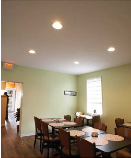
BEFORE: Plaster ceiling
