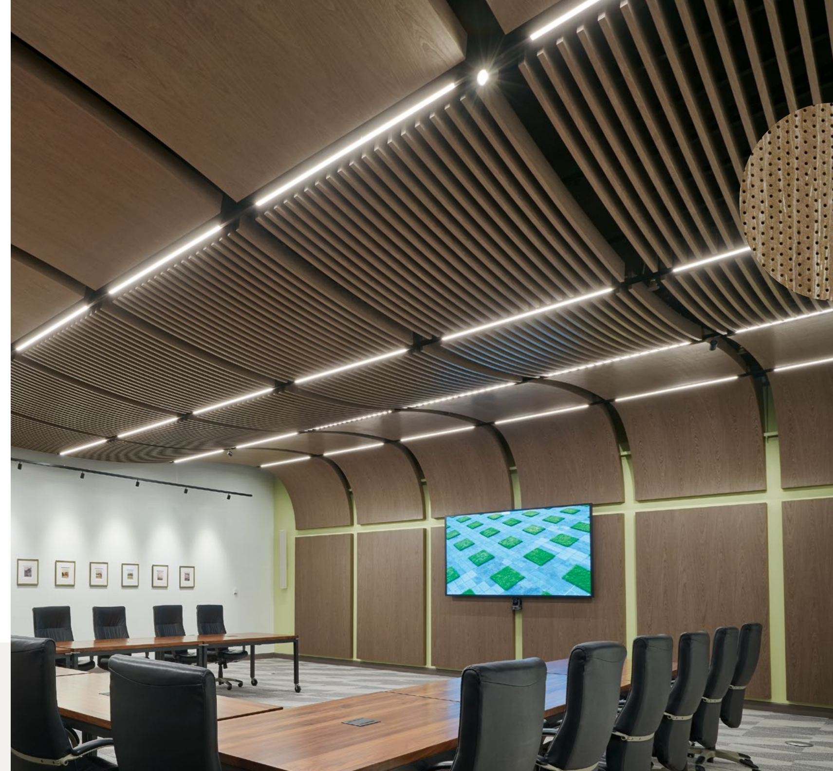
Custom WoodWorks® micro-perforated ceiling and wall panels
