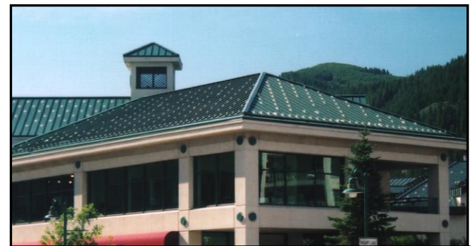
Figure 8B: “Cleat” type snowguard system
