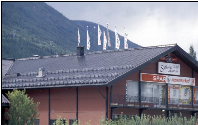
Figure 9: This project in Norway demonstrates appropriate placement of multiple rows, concentrated in the lower half of the roof
