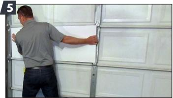
Insert the panel (laminated side facing outward) under one horizontal rail, carefully bending it in order to place the other side behind the opposite rail.
