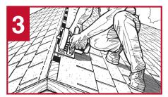
Cut along chalk lines. Remove roof sheathing. **Note:** Slot should not be cut any closer than within twelve (12) inches of gable end, hip intersecting ridge.
