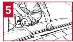
Nail each additional section in the same manner until entire ridge is covered. A chalk line may be utilized to ensure vent alignment. Cut last piece to length and install with original uncut end to the outside.
