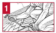
Remove ridge cap shingles from the entire length of the ridge. **Note:** Delete Step 1 for new construction.
