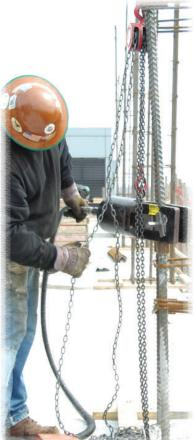
BarGrip XL cold–swaged coupling sleeves consist of seamless steel sleeves that slip over the ends of reinforcing bars. They are swaged onto the reinforcing bar profile to produce mechanical interlock.
