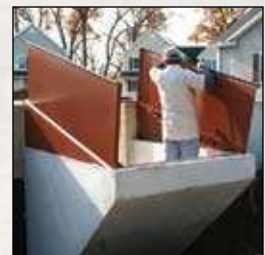
4. The Bilco door is assembled and anchored to the precast stairwell. The area is then backfilled and landscaped to complete the installation.
