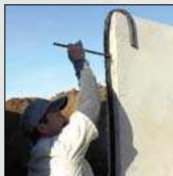
2. Facing surfaces are coated with self-sealing butyl resin strip sealant for a watertight seal and rods are threaded into anchors built into the casting.
