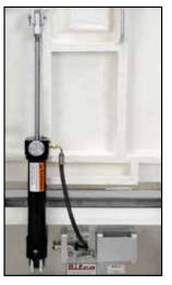
Self-closing mechanism Automatically closes the door in the event of a fire. Door remains firmly closed to prevent the spread of fire between building floors.
