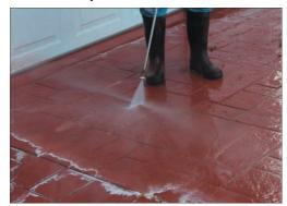
It is vital to make sure the surface is clean and ready to accept pigment. The surface should be free of sealers, dirt, oil, grease, dust, and other contaminants. Furthermore, the concrete should be porous and ready to accept the Antique-It. Use a cleaning and etching agent, such as BRICKFORM E-Etch, to properly prepare the surface.
