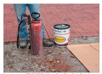
Apply a sealer (BRICKFORM Gem-Seal, Poly-Seal, Poly-Astic, DecoPoxy, or UreMax) as soon as possible. Allowing traffic on the surface before it is sealed can deteriorate the Antiqued finish or introduce contaminants that will affect the sealer's coverage.
