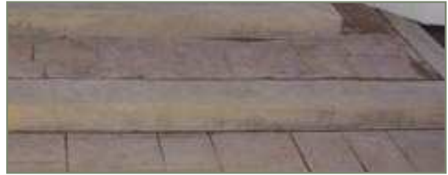
Before old, discolored concrete
