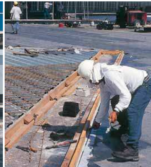
While applicators are busy coating one segment of the concrete roof, a worker lays down a coat of primer with an airless sprayer on another section (above left). Elsewhere, a worker applies caulking to a vertical transition that will become part of a raised planter (above right).
