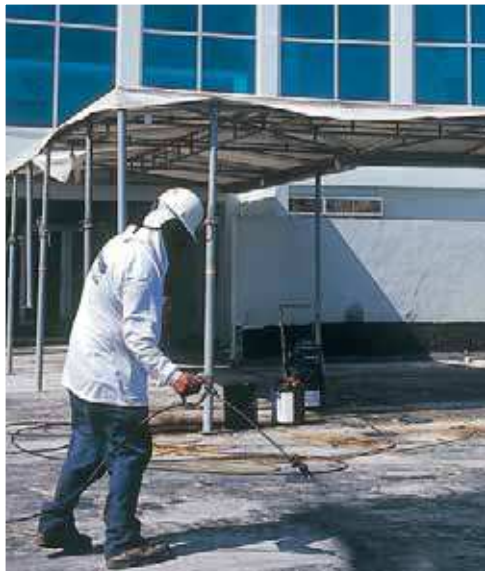
While applicators are busy coating one segment of the concrete roof, a worker lays down a coat of primer with an airless sprayer on another section (above left). Elsewhere, a worker applies caulking to a vertical transition that will become part of a raised planter (above right).
