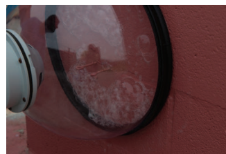
Coating B – Brick Tie Condition Air Leakage (Bubbles) Through Pores
