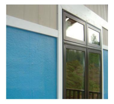
OSB construction with fiber cement siding nailed directly over the sheathing. Thicker membrane consistently covers rough, absorbent OSB surface while sealing around penetrations and providing continuity over edges of window flashing and sheathing joint reinforcement.
