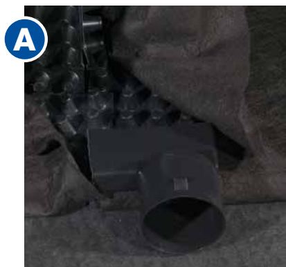
6" Endout Connector attached to CCW MiraDRAIN HC
