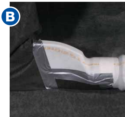
CCW MiraDRAIN HC Connector attached to end of CCW MiraDRAIN HC & covered with extra filter fabric on cut edge and adhered with tape
