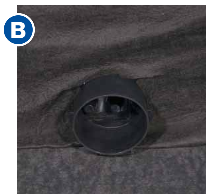
6" Sideout Connector covered with fabric
