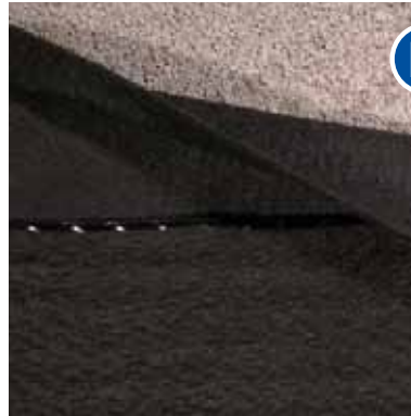
A Cut approximately 3" (75 mm) of core leaving the geotextile fabric to overlap the adjacent panel. The fabric can be adhered with approved CCW adhesive. (Optional: Cover butted core with additional geotextile fabric.)
