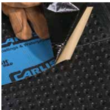
CCW MiraDRAIN joined top-to-bottom with 4" CCW-705
