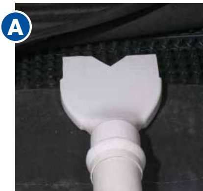
CCW MiraDRAIN HC Connector attached to side of CCW MiraDRAIN HC
