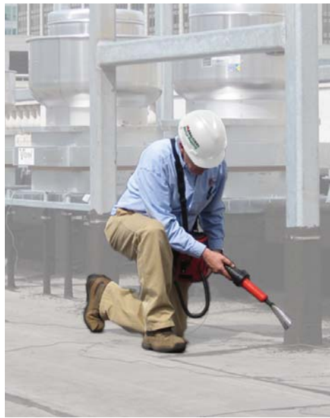
High-Voltage Electronic Leak Detection
