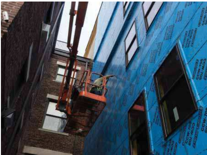
CCW-705 Air & Vapor Barrier Strips Application.
