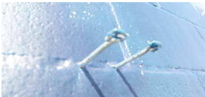
Fire Resist Barritech NP60 cured membrane over CMU.
