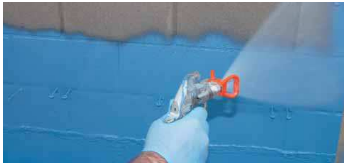
Spray application of Fire Resist Barritech NP60.
