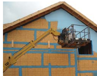
Fire Resist Barritech VP sprayed over joint details
