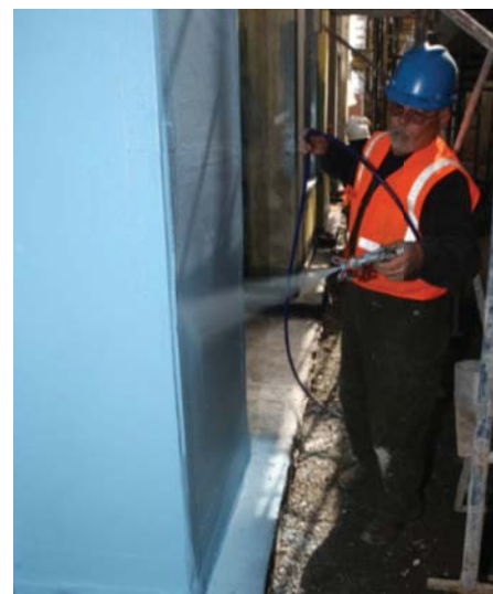
Fire Resist Barritech VP spray application.
