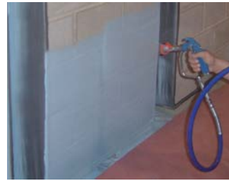
Fire Resist Barritech VP spray-applied in a single coat at 60 mils wet on concrete block
