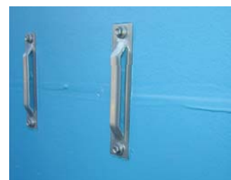
Installed using screws with neoprene washers
