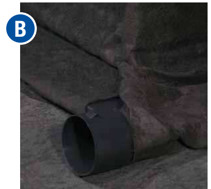
6" Endout Connector covered with fabric
