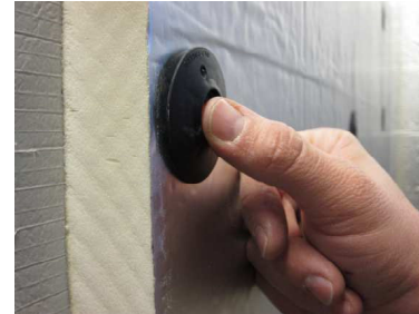
Pre-spot washer on insulation.
