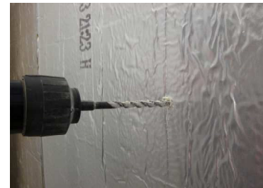
1. Drill through insulation and into substrate with 5/16" masonry bit
