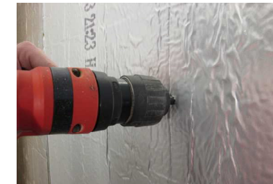
1. Drill through insulation and into substrate with 5/16" masonry bit
