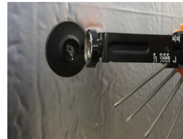
Drive screw until secure. Washer flattens on surface of insulation.
