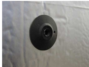
Pre-spot prongs into surface of insulation for easy screw assembly.
