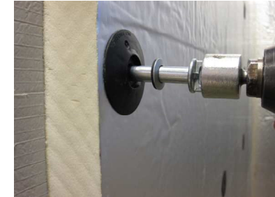
Insert brick-tie into chuck.
