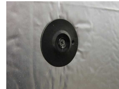
Drive screw until secure. Washer flattens on surface of insulation.
