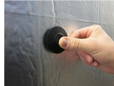
1. Pre-spot Thermal-Grip® ci washers on insulation surface
