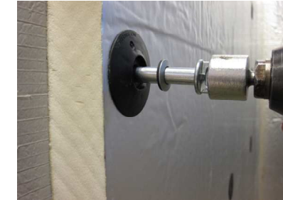
Insert brick-tie into chuck.
