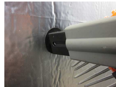
3. Drill gun screws to pre-determined depth preventing overdrive
