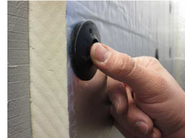
Pre-spot washer on insulation.
