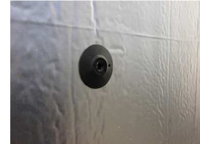
1. Pre-spot Thermal-Grip® ci washers on insulation surface
