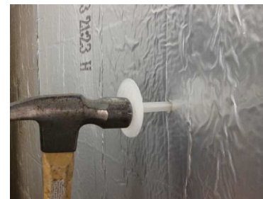
3. Tap with hammer until head is flush with insulation surface
