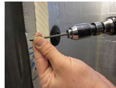
2. Insert Grip-Deck® screw (sds or coarse) into EZ-Driver
