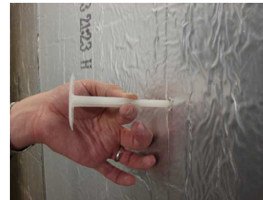
2. Insert Plasti-Grip® PMF into drilled hole
