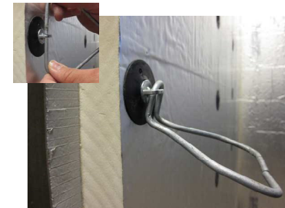
Attach wire-tie for masonry veneer.
