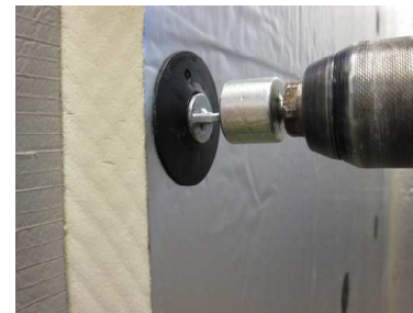
Fasten brick-tie securely.
