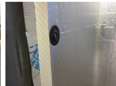
4. EZ-Driver releases fastener at preset depth preventing overdrive
