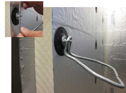
Attach wire-tie for masonry veneer.
