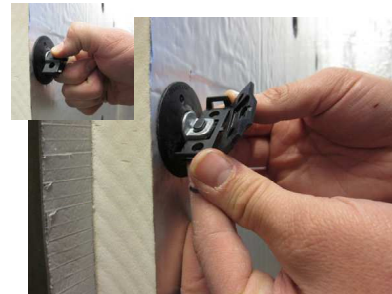
Thermal-Clip can be added for added thermal-break (from Heckmann).
