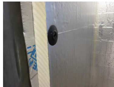
1. Pre-spot Thermal-Grip® ci prong washers on insulation surface
