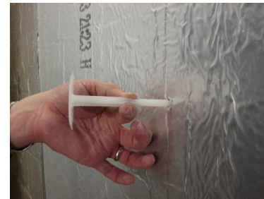
2. Insert Plasti-Grip® PMF into drilled hole
