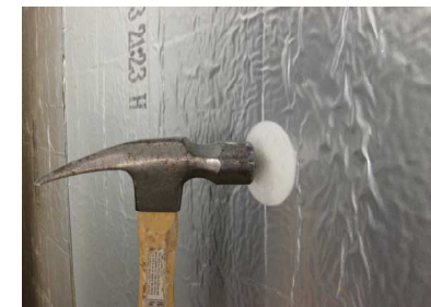
3. Tap with hammer until head is flush with insulation surface
