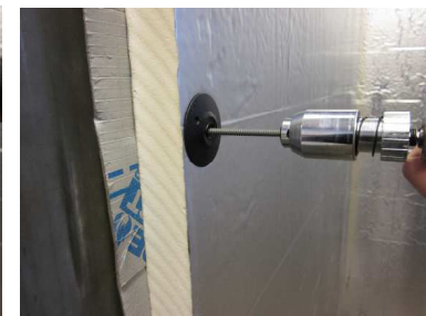
2. Insert Grip-Deck® screw (sds or coarse) into EZ-Driver
