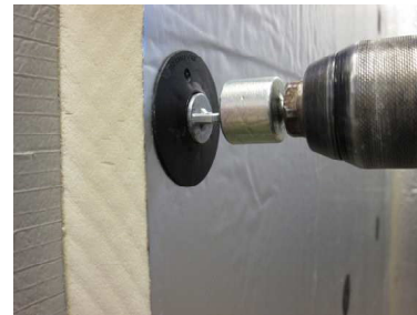
Fasten brick-tie securely.
