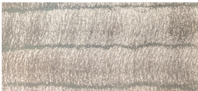
Proper Coverage on Insulation
