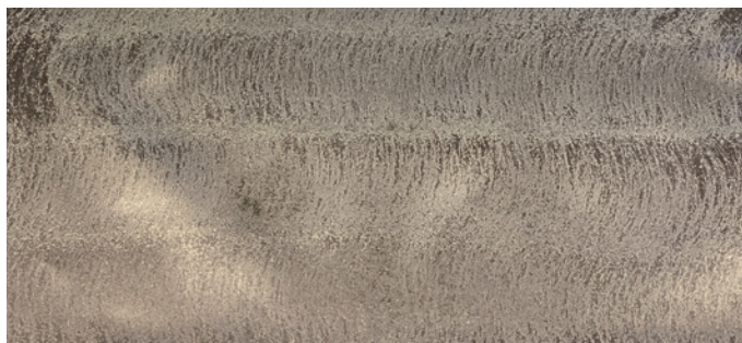
Proper Coverage on Membrane
