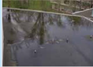
Flooded roof due to improperly designed taper.
