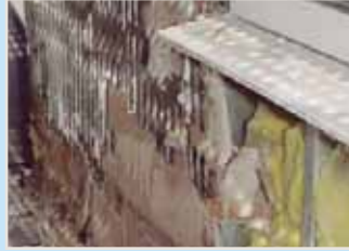
This deterioration was caused by lack of waterproofing in window openings.
