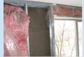
Condensation in wall insulation from air leakage.
