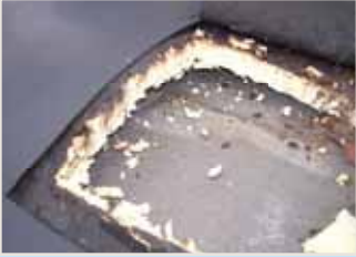
Moisture infiltration caused the insulation to deteriorate and the fastener to rust, putting the roof at risk of blowing off.
